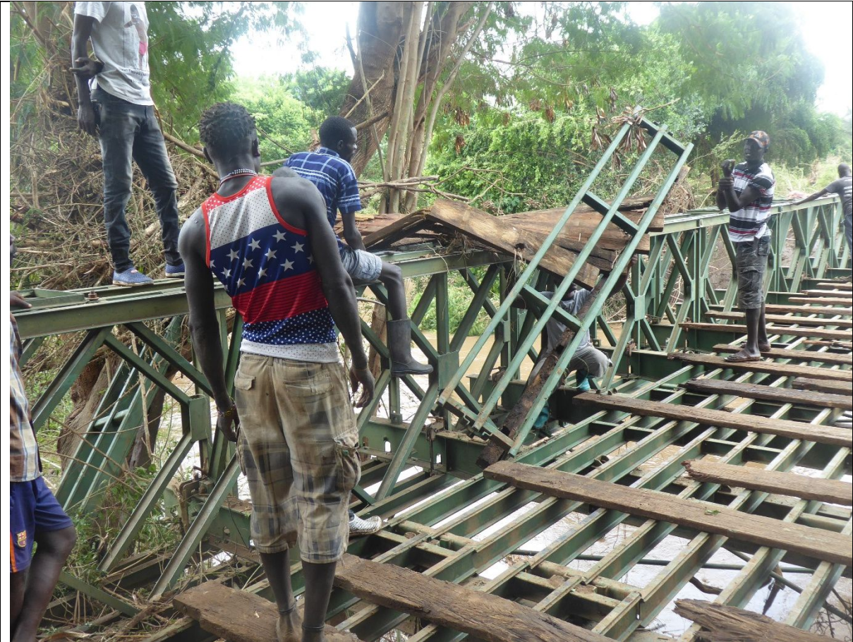
The motor bridge in Kuron under rebuilding
